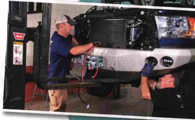
Truck Supply & Outfitters fits our Crew Cab Ram with a Road Armor Bumper/Warn winch combo.
